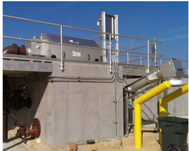
Perforated Plate Drum Screen Used to Protect Integrity of the Media and Improve Biological Process Efficiency
