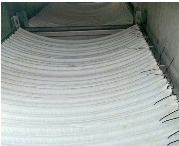
Fixed Hydrophilic Textile Nylon Media Unit that is used to Attach the Biofilm
