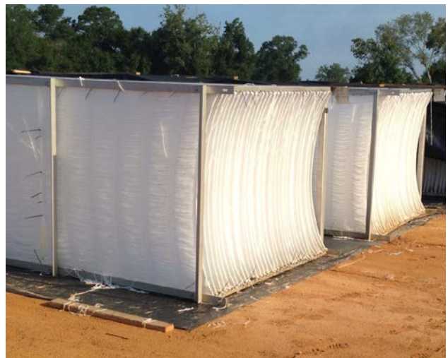
Fixed Hydrophilic Textile Nylon Media Unit that is used to Attach the Biofilm
