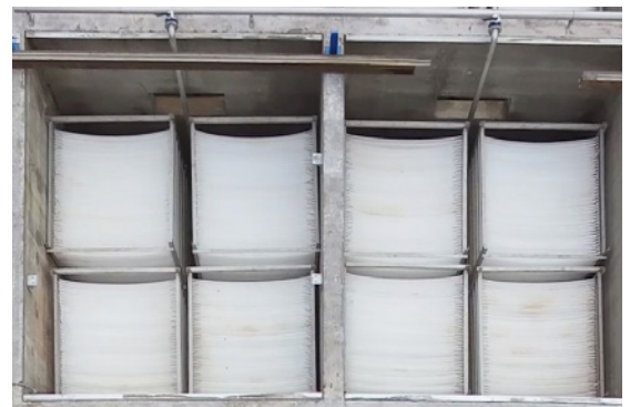
Nebula Biofilm Media Installation
