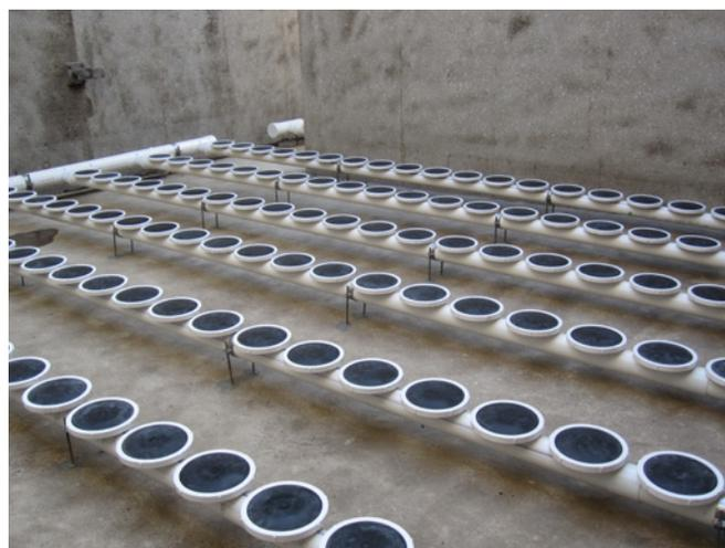
Quantaer Fine Bubble Disc Diffuser System
