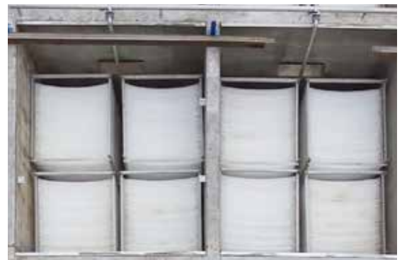
Nebula Biofilm Media Installation
