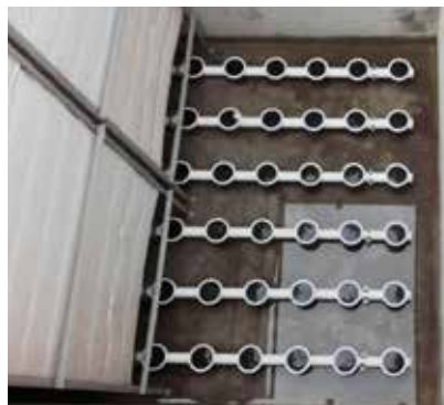
Quantaer Fine Bubble Aeration System
