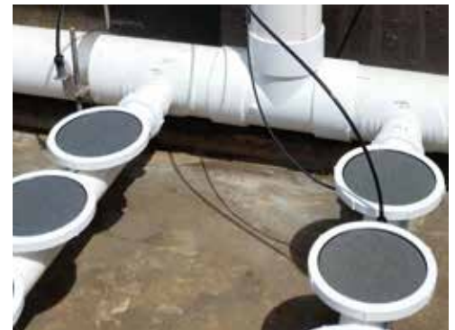
Cleaning and Monitoring System
