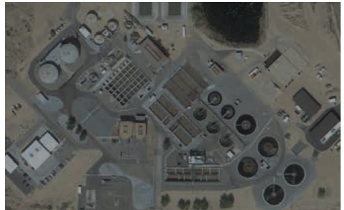
Victor Valley Wastewater Reclamation Authority, California
