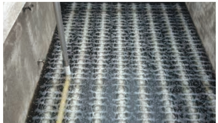
Quantaer EPDM Membrane Disc Diffusers Operating at Startup
