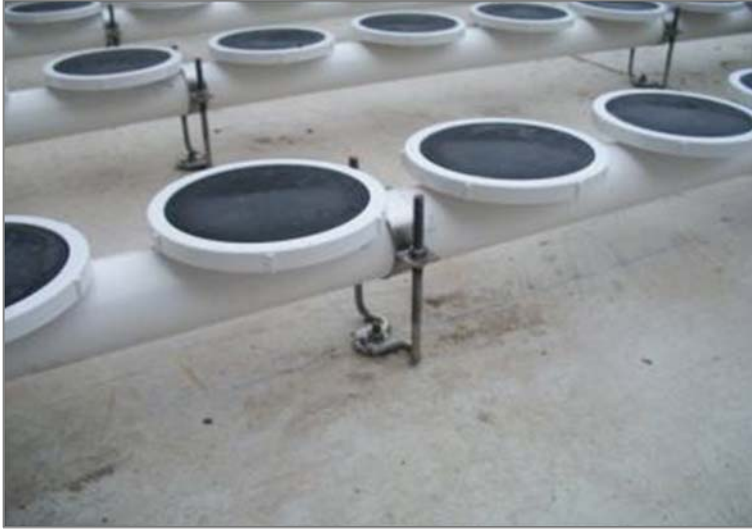
Air Distributors and Supports Installed
