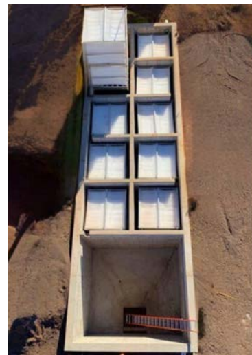
The ten treatment stages and final clarifier provide improved secondary treatment, integrating perfectly with existing plant infrastructure.
