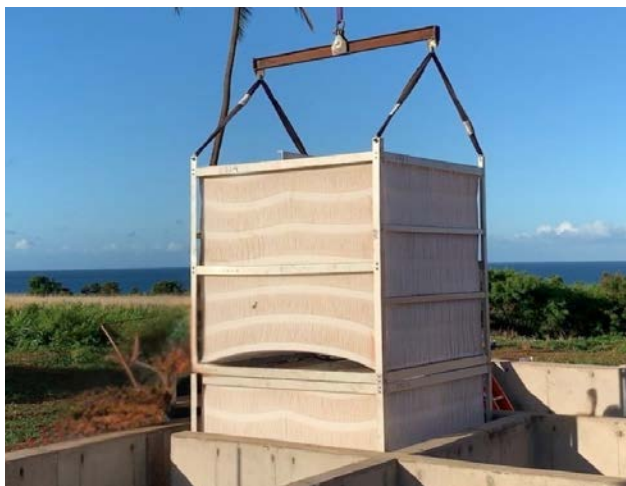
Ten media racks were installed, one per treatment stage. The media provides an ideal growth surface for the discrete microbial populations driving treatment.
