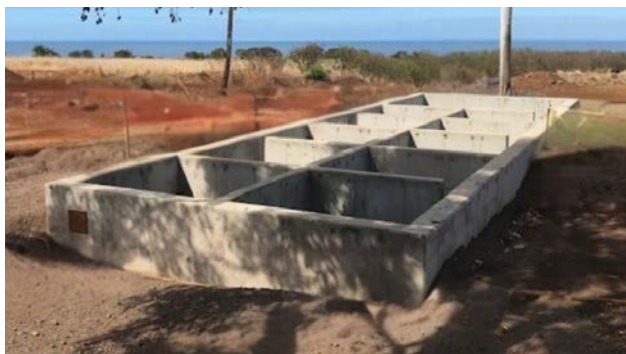
The baffles inside the basin allow for a plug flow through isolated zones of treatment—the key to establishing the microbial food chain responsible for sludge reduction.
